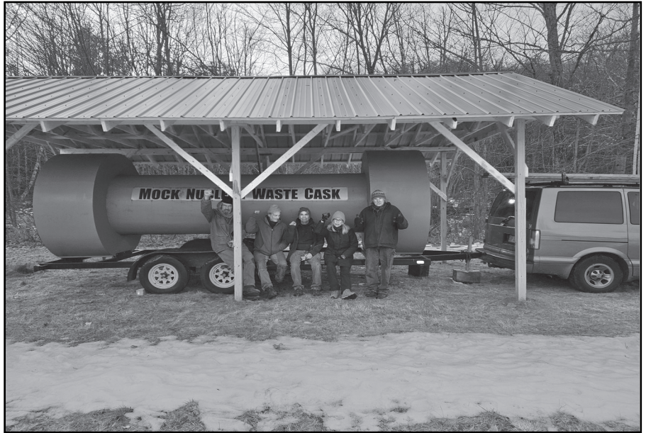
The completed storage shed for CAN's Mock Nuclear Waste Cask
