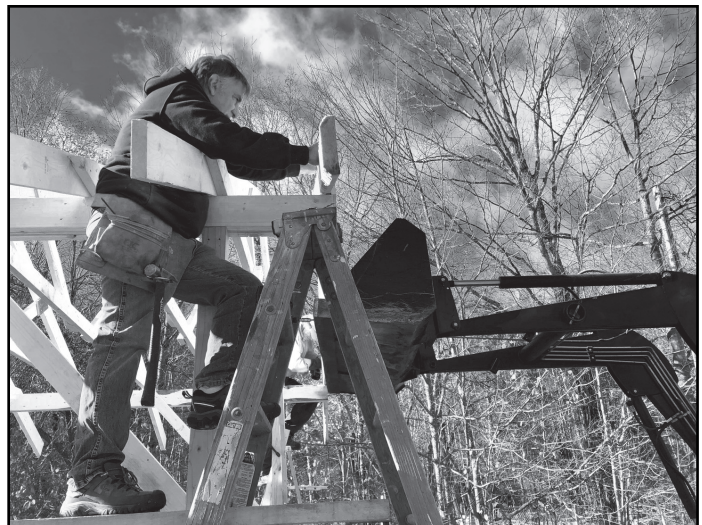
Bob Bady working on the roof of the shed
